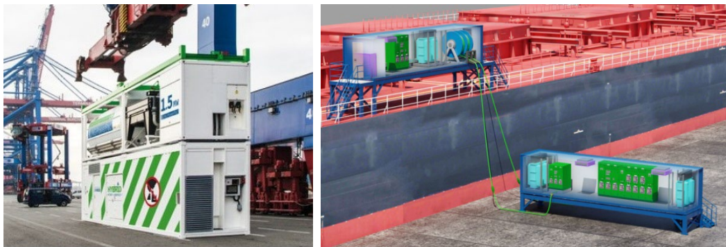
Fig.2d. Container-based OPS systems (normally in high-cube containers).
